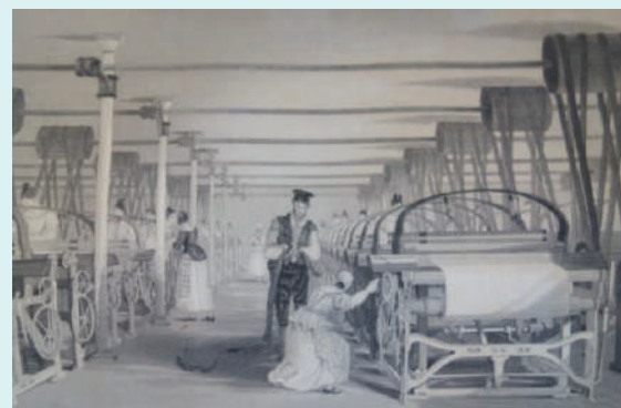
Power loom in a factory 28
